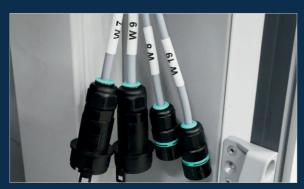
Prepared and encoded connectors for easy cabling.
